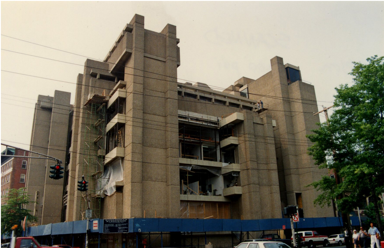
Exterior of Rudolph's Yale School of Architecture under renovation. Photo by Zak Ghanim.
